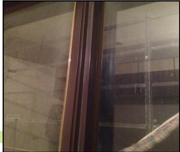
Figure 1: Slit between the window slides
